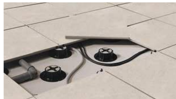
Laying as raised paving. Colocación sobreelevado.
